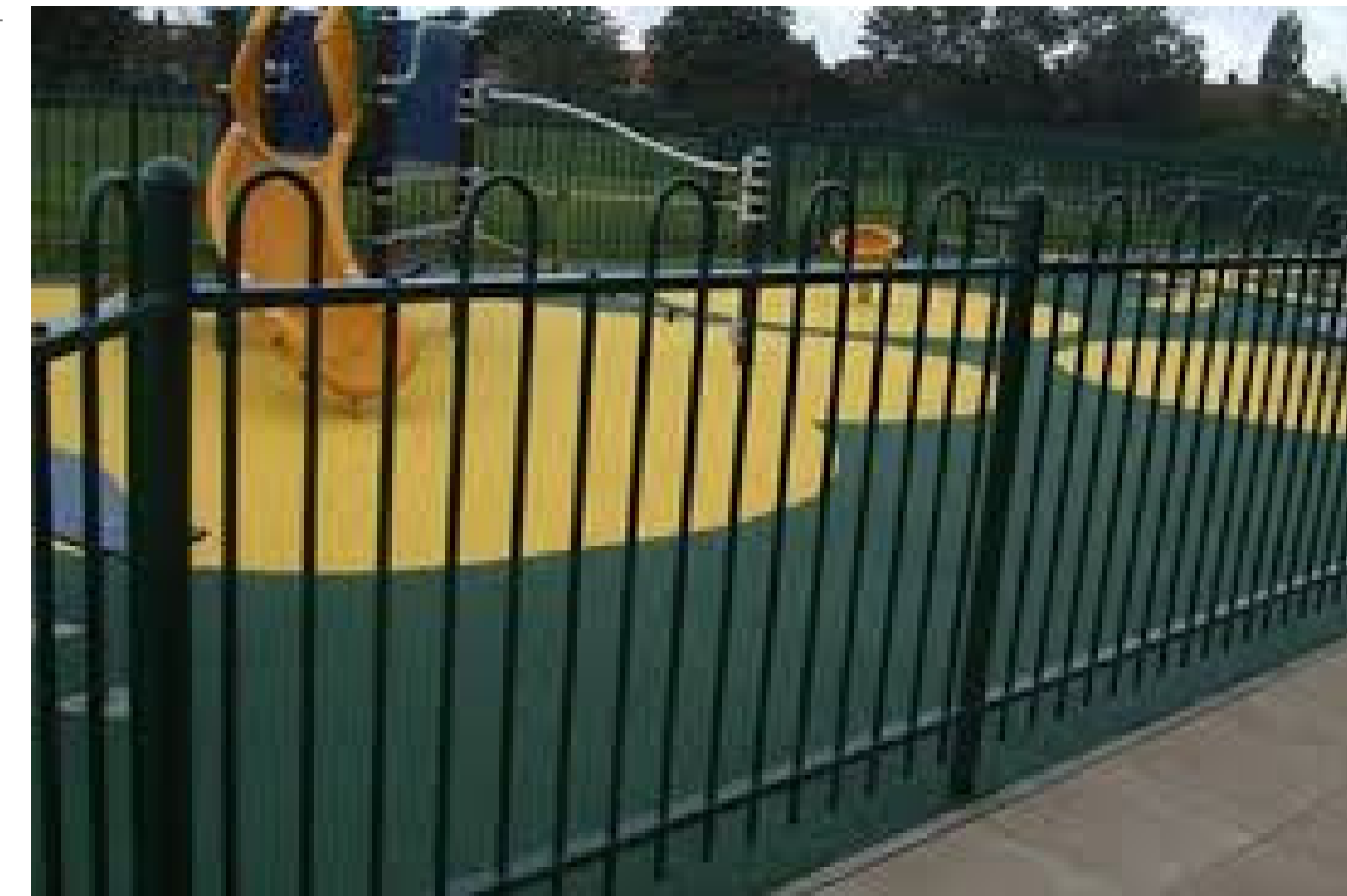
Bow Top Safety Fencing around LEAP
