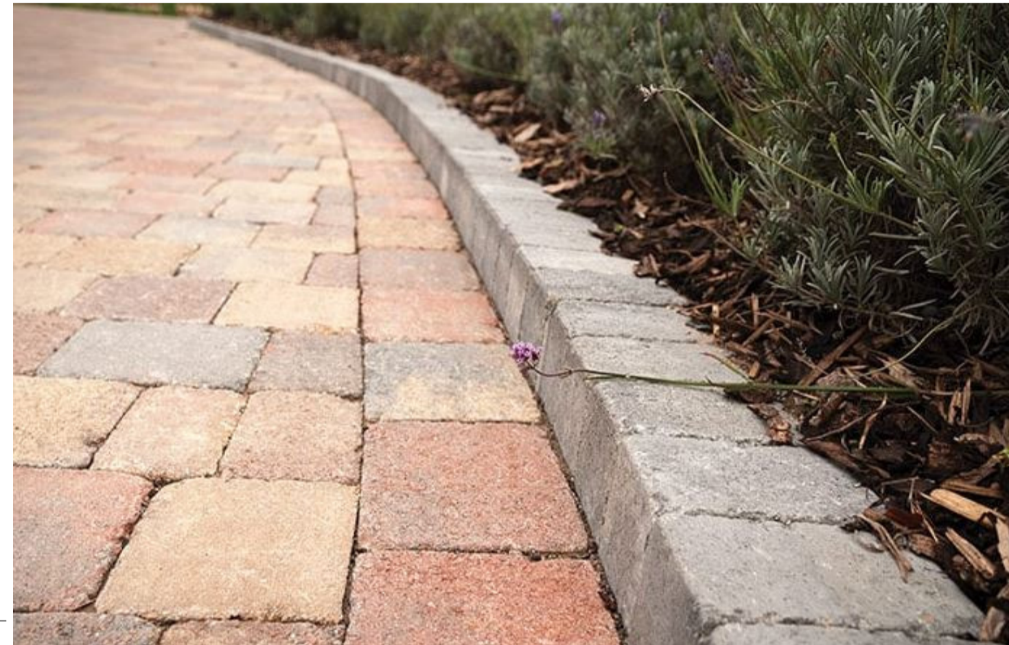
Hydropave Private Drive Surface and Kerb
